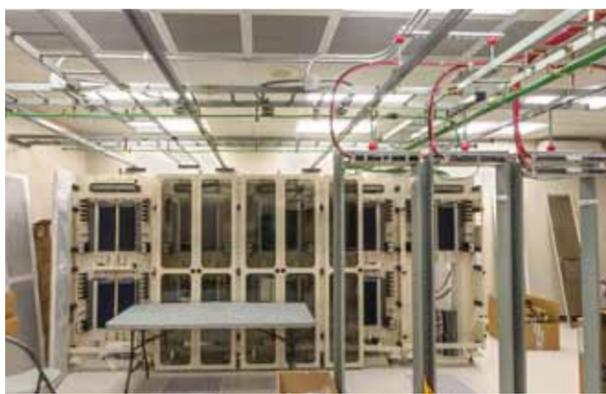
*fiber distribution frames terminating close to 6000 fibers*
